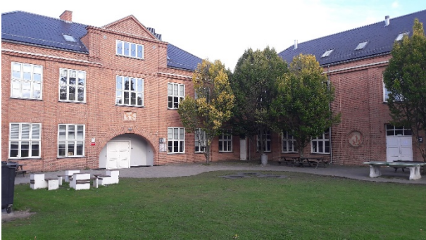
Figure 3. Facade of the building of the school.
