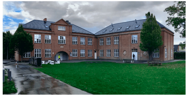
Fig. 1. A photograph of the building site.
